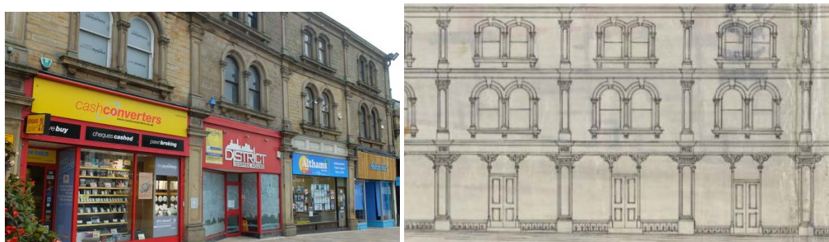
Figure 6: Example shown here is Virgil Andertons Shops, Nos 4-14 St James Street, built c.1876, Listed Grade II. Note the original shopfronts have been replaced by ones that are poorly designed and poorly related to the period, style and overall composition of the building facade in terms of their mixed framework, proportions, materials and detailing particularly fascias, signage and colours. Any replacement shopfronts should be designed to achieve a degree of uniformity in design and proportion.
