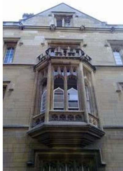
Figure 3: Left - A late Georgian shopfront with earlier styled bowed oriel windows, Kirby Lonsdale. Right: Ornate canted oriel window (oriel windows project from the plane of the building but don't touch the floor like full bay windows do).
