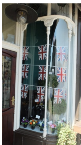
Figure 8: Well preserved surviving early Edwardian shopfront in Padiham. Note the slender mullions and transoms, leaded and stained glass detailing to the transom lights, curved glazing to recessed doorway with mosaic tile threshold.
