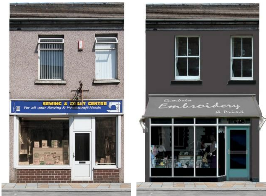
Figure 14: How modern shopfronts on a traditional buildings might be improved using appropriate traditional and contemporary detailing
