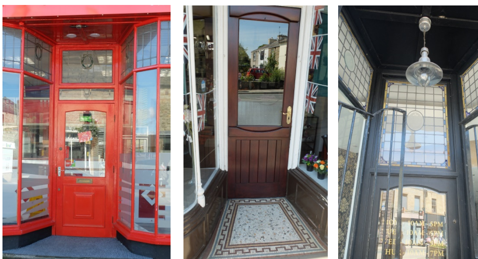
Figure 23: (Left) Traditional doors were glazed with a kick plate at the bottom typically at the same height as the adjoining stallriser, and with a window above the door frame called a fanlight (Middle) recessed doorway with flanking windows and tiled threshold (Right) Leaded fan-light
