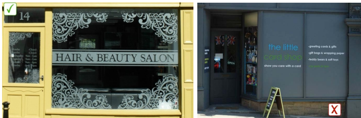
Figure 28: (Left) The use of carefully designed etched window stickers sensitively applied to the window can improve the appearance of a shopfront whilst also maintaining views inside. (Right) The shopfront window is completely obscured by signage creating an oppressive and unwelcoming shopfront.
