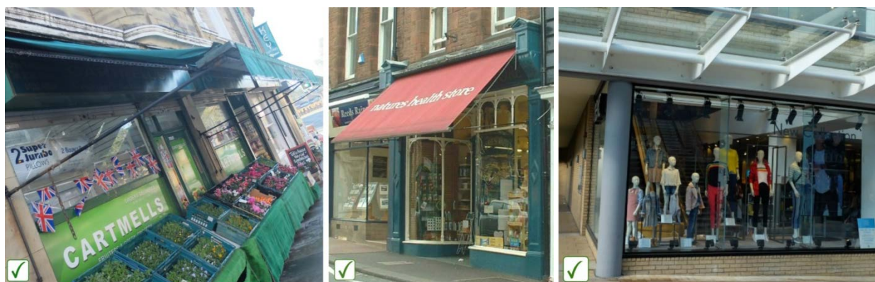
Figure 33: Left: A traditional retractable canvas blind, metal arms extend out and storm chains prevent excessive movement. Centre: An attractive & well-maintained traditional shopfront with fully-retractable canvas blind with the blind box located below within the cornice. Right: Cantilevered glass canopy to a modern shopfront in Burnley Town Centre.
