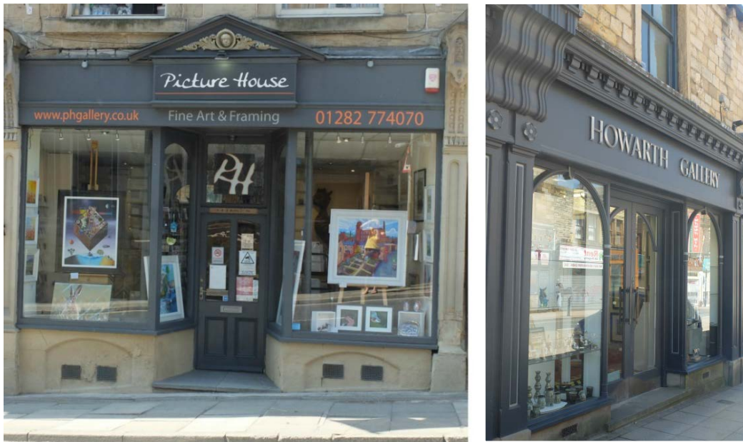
Figure 13: Traditional shopfront design incorporating elements such as transom windows, decorative pilasters and corbels. Features such as these give traditional shopfronts a strong sense of character as a result of these being more decorative and detailed than modern approaches. These are not an original shopfronts, but are attractive, and well-constructed traditionally-styled shopfronts appropriate to the style and character of the buildings.
