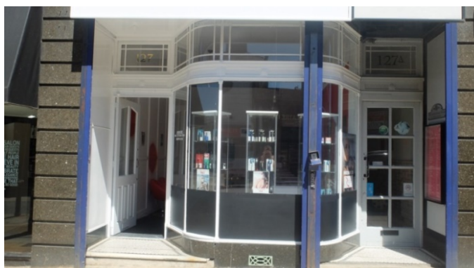
Figure 9: Attractive 1930s recessed shopfront at the Empire Buildings, No. 127 St James Street. Note the deeply recessed and tiled lobbies, curved glass, etched fanlights, shallow stallriser, decorative vents and marble pilasters.
