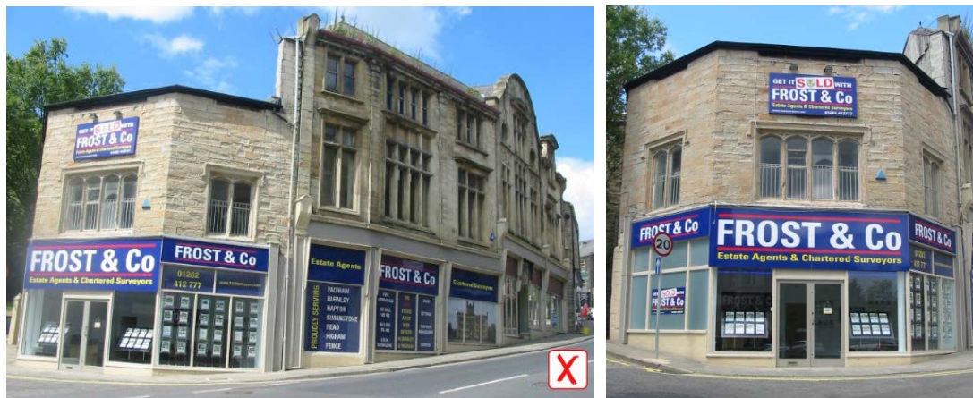
Figure 29: Examples of the visual clutter caused by an overbearing fascia, poorly designed and poorly located signage, posters and window graphics.
