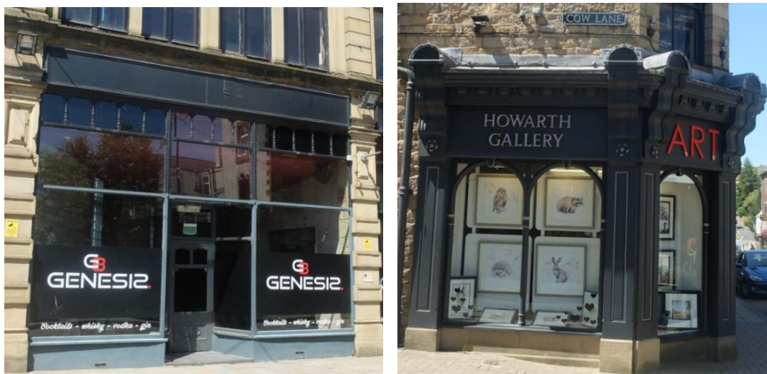
Figure 5: Restored late Victorian styled shopfront at the former Burnley Co-operative Society Premises, Hammerton Street Burnley (left) and Victorian styled shopfront with modern lettering, St James Street (Right).
