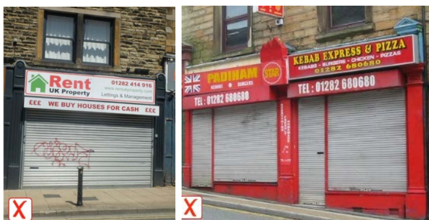
Figure 34: Solid shutters prevent visibility into the shop outside operating hours together with their associated guide-rails and boxes can spoil the appearance of a building and adversely affect the appearance of an area under threat, thus inviting further damage.
