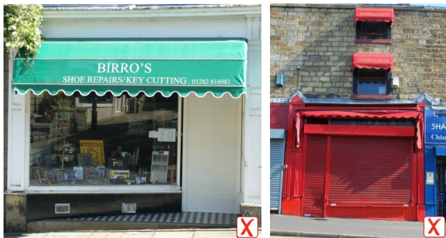
Figure 32: (Left) An example of a fixed Dutch style canopy blind and (Right) Modern folding 'fan' blinds are difficult to recess in an acceptable manner
