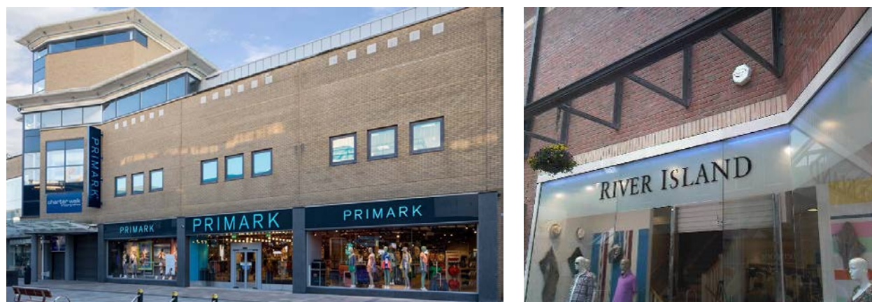
Figure 17: (Left) Modern shopfront on a modern building in Burnley Town Centre. A traditionally styled shopfront would not necessary in this context. (Right) Modern frameless glazed shopfront in Cumbria
