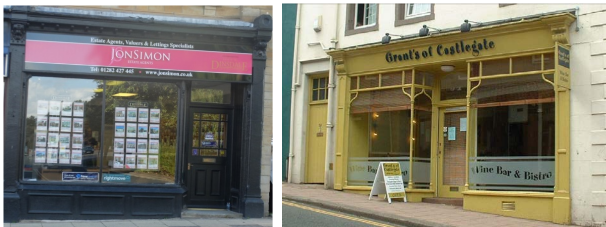
Figure 25: Left: A high quality Victorian shopfront, but the traditional detailing is somewhat lost by the single dark colour used and the quality diluted by the acrylic fascia sign extending over what may have originally been transom lights. Right: The contemporary colour scheme, signage and styling of this shopfront in Cumbria shows how a modern business can successfully utilise a traditional shopfront
