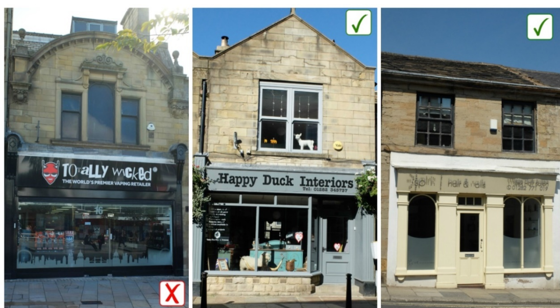
Figure 19: (Left) Flat shopfront insert and undivided glazing detracts from the existing traditional frame and the character and appearance of the host building. (Middle and Right) Recessed doorway and projecting cornice and corbels project light and shadow over shopfronts.
