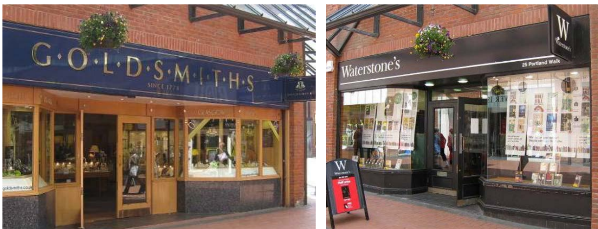
Figure 16: Examples of attractive and well-presented modern interpretation of traditional shopfronts (Cumbria). Left: A more traditional and elaborate timber detailing to this modern shopfront. Right: A predominantly timber shopfront with modern frameless glazing but with profiling to the timberwork adding dimension, and sitting within the building's brick piers which provide framing, separation and solidity.
