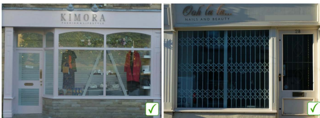
Figure 37: Left: This internal shutter coupled with good internal lighting allows for a window display to be maintained, adds life to the street and allows window shopping outside of opening hours. Right: Retractable internal lattice gate type shutters also allows view into the (lit) shop
