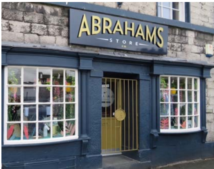
Figure 3: Left - A late Georgian shopfront with earlier styled bowed oriel windows, Kirby Lonsdale. Right: Ornate canted oriel window (oriel windows project from the plane of the building but don't touch the floor like full bay windows do).
