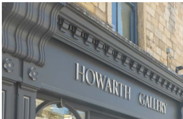
Figure 22: A reproduction of a traditional style fascia and cornice
